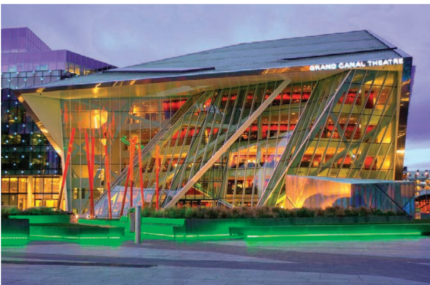
Photograph Courtesy of Kalzip
