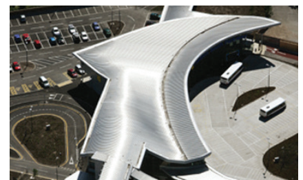
Photograph courtesy of Kalzip
