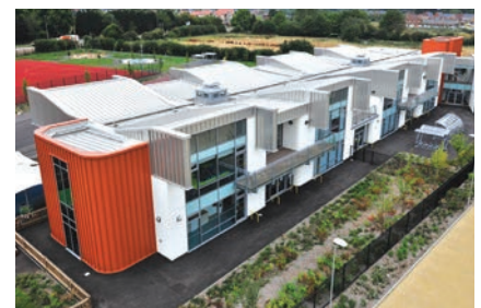
Photograph courtesy of Kalzip
